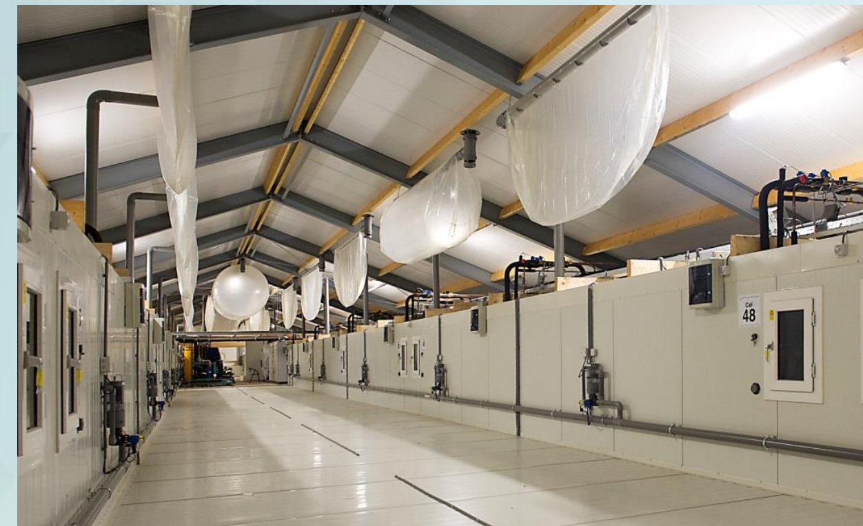
e. Cooling controlled area above CA rooms & corridor. Dust & oxidation free to protect all technical installations. Easy to access.
