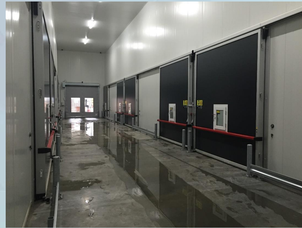
c. CA rooms and cooled corridor & equipment area on top
