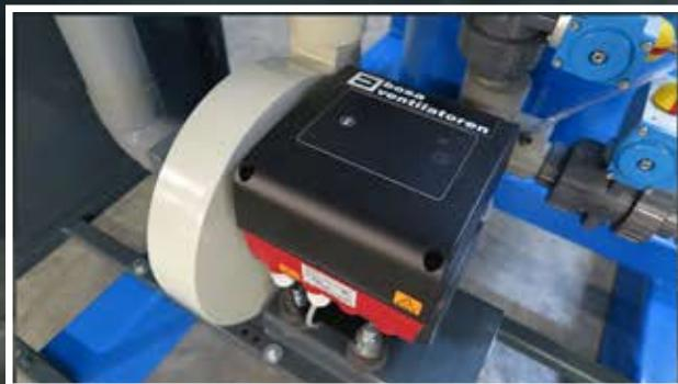
Frequency controlled motor, low energy consumption and limited starting current. This is possible because this motor is directly driven and does not use a V-belt
