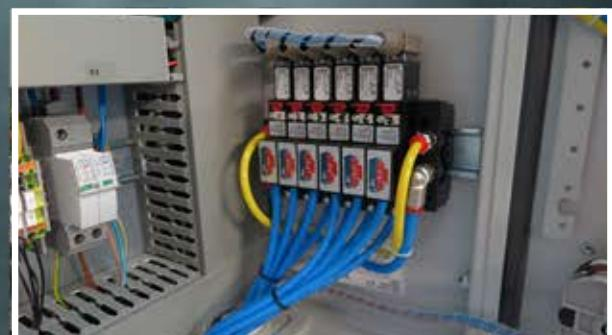
High-quality Burkert valves for controlling butterfly valves. This improves the reliability of the system so that the machine remains low in maintenance
