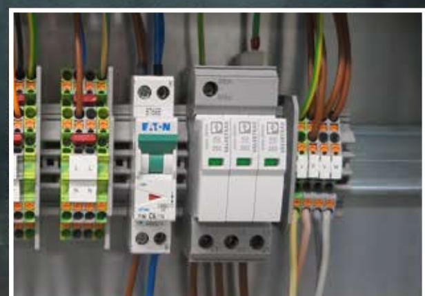
All our CO<sub>2</sub> Adsorbers are standard equipped with an overvoltage protection to protect the fan. In this way, the fan will never be damaged when for whatever reason it has to deal with overvoltage
