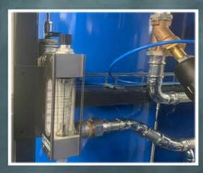
The flow indicator on the outlet side has a manually adjustable valve to adjust the flow. You can read the flow by the level of the floater in the transparent tube
